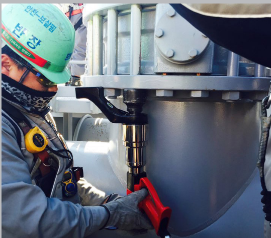
Daewoo Engineer performing bolting task on flange
